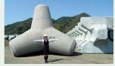
Large breakwater blocks (20–80t) at a nuclear power station are made with coal ash produced at coal-fired thermal generating stations.
